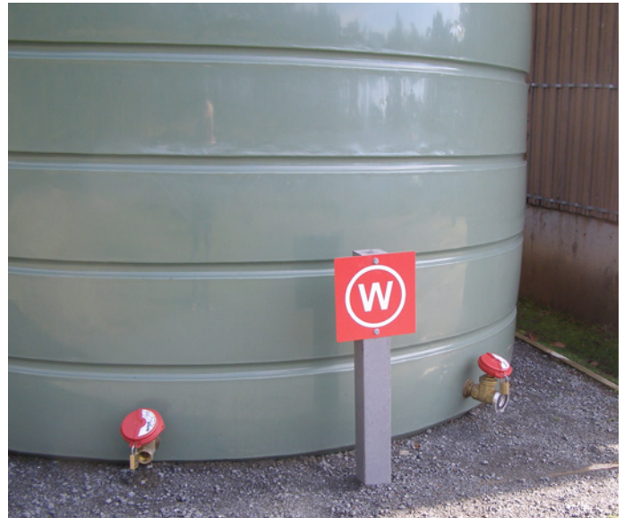
An example of how the water tank sign should be placed
