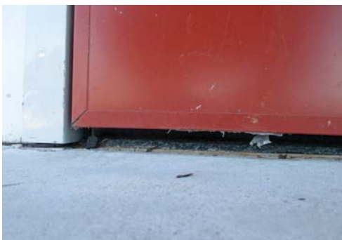
Figure 3: Window and door gaps
