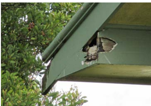
Figure 4: Damage and decay
