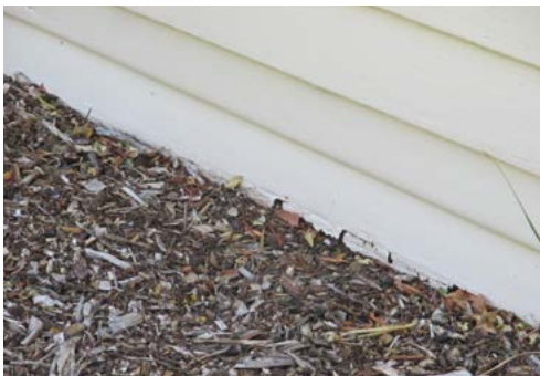
Figure 6: Mulch close to buildings
