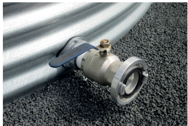
Figure 3 A water connection point with Storz coupling
